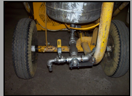
All New Stainless Steel Lower Plumbing
